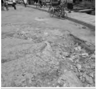
Plate 1.3: Eroded Drop Off (Kakamega)
